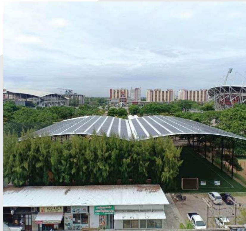
Flick TU 251.10 kWp
