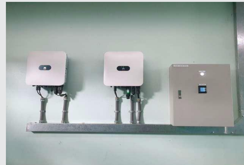
Installation example inverter
