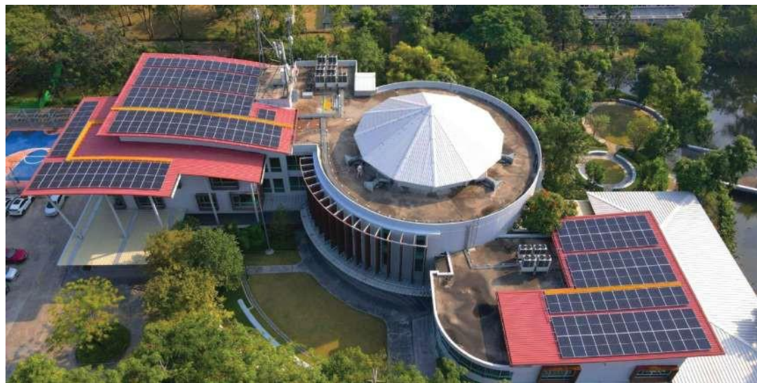
Puey Ungphakorn School of Development Studies 117.72 kWp
