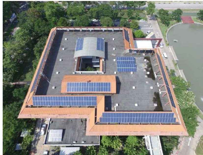
Office of the President 111.60 kWp
