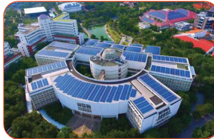
Solar Rooftop System 30 MW
