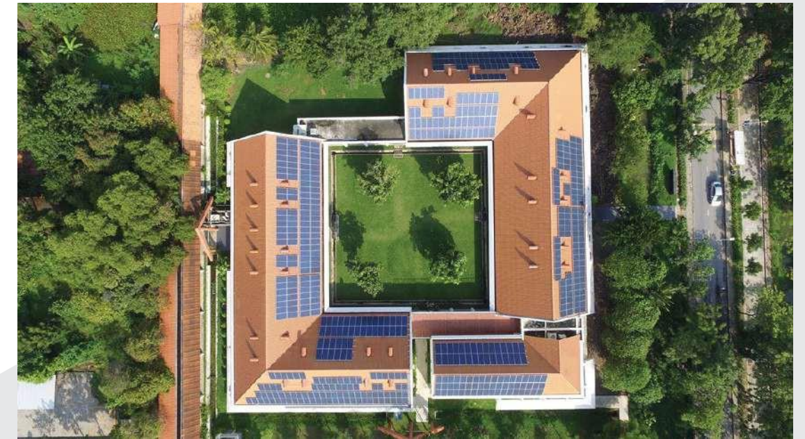
Academic Building 133.92 kWp
