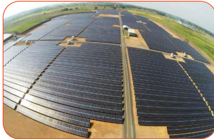
EPC to Power Plant 155 MW
