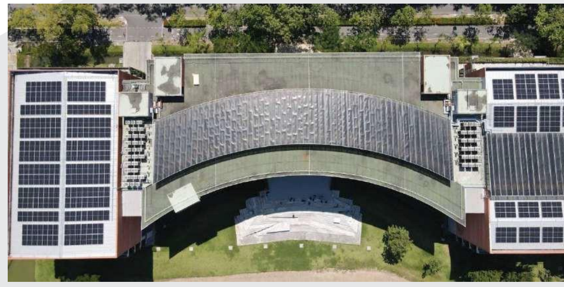
SC3 Building 470.88 kWp
